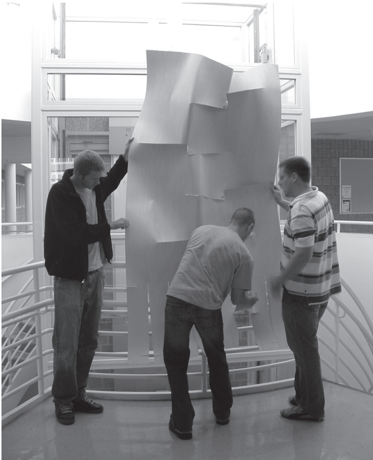
INSTALLING VENEER PANEL
